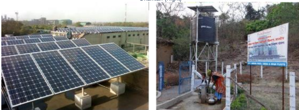
Figure 36: 100 KW SPV Power Plant Installed at SEML, Siltara, Raipur (Left) Solar Drinking Water Pump at Siyarinali, Dist. Dhamtari (Right)
