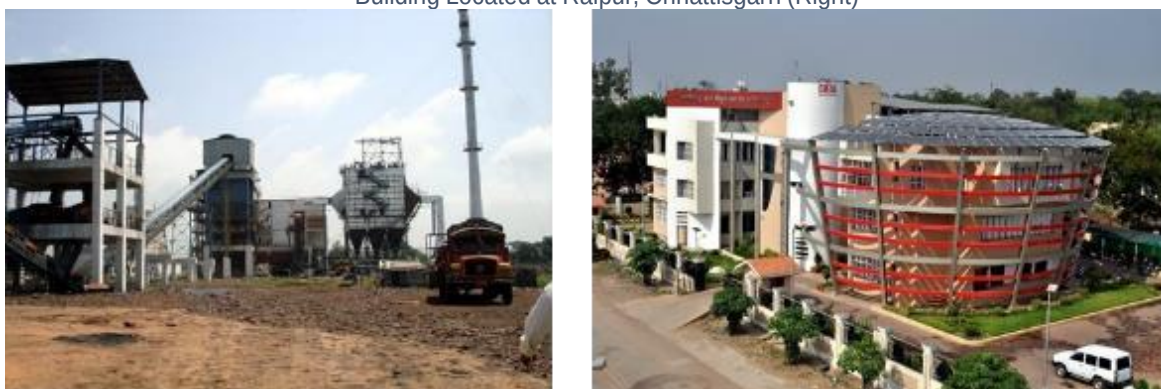
Figure 37: Biomass Gasifier Installed at, Vill Banki, Block Bodla, Dist. Kawardha (Left) CREDA Building: 1st Energy Plus Building Located at Raipur, Chhattisgarh (Right)
